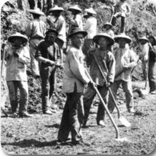
Chinese laborers working on a railroad in California.
