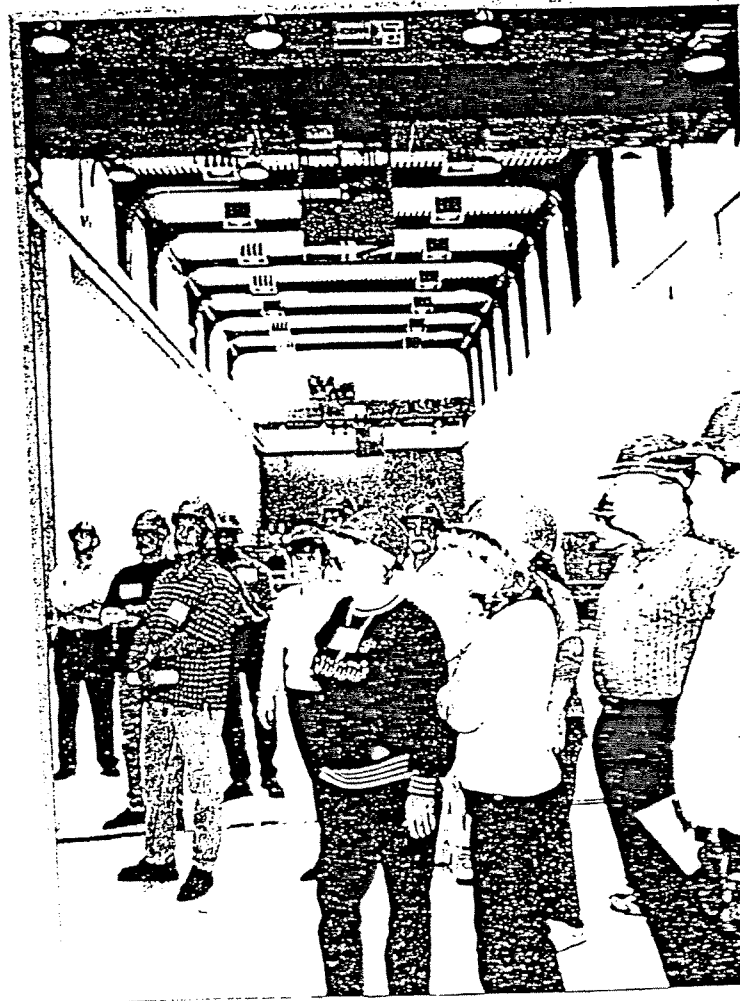
At Edmonston Pumping Plant (at the base of the Grapevine), State Water Project Inspection Trip guests learned how water is pumped up 2,000 feet to travel.
