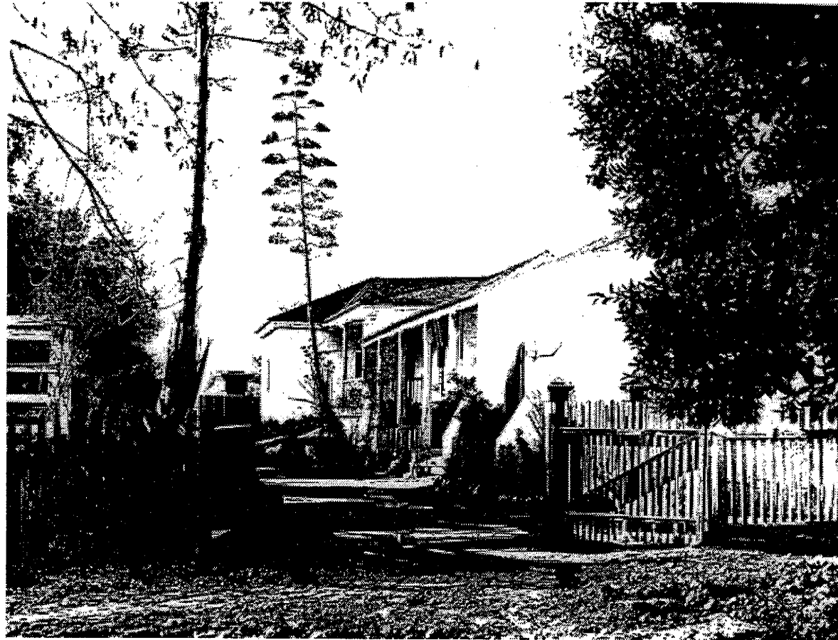
View of Ygnacio del Valle adobe from Southeast entry of original drive. Note the arbor at left and the white picket fence.
