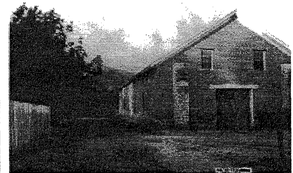
The Winery, as it appeared at the turn of the century. Note the picket fence along the drive.
