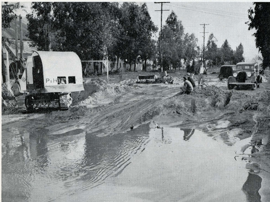
This is how flood left E Street in San Bernardino, a thoroughfare leading to famous Orange Show Pavilion, which can be seen on the left of power shovel removing five feet of mud.
