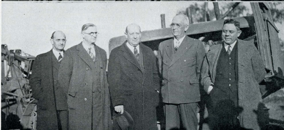
Scenes at groundbreaking on Arroyo Seco Highway. Upper—Miss Cheryl Walker moves first earth with huge tractor. Lower—Left to right: John C. Jacobs, mayor of South Pasadena; Arthur Kennedy, president Los Angeles City Planning Commission; Roger W. Jessup, chairman Los Angeles Board of Supervisors; E. O. Nay, president Board of City Commissioners, Pasadena; Harry A. Hopkins, Assistant State Director of Public Works.
