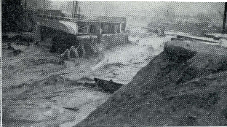
Before and after views of the bridge across Verdugo Creek on State Highway 61 in Los Angeles County. Fed by small tributary streams in the San Gabriel Mountains the creek became a raging torrent that cut a new channel, swept away the bridge approach and damaged the abutment.
