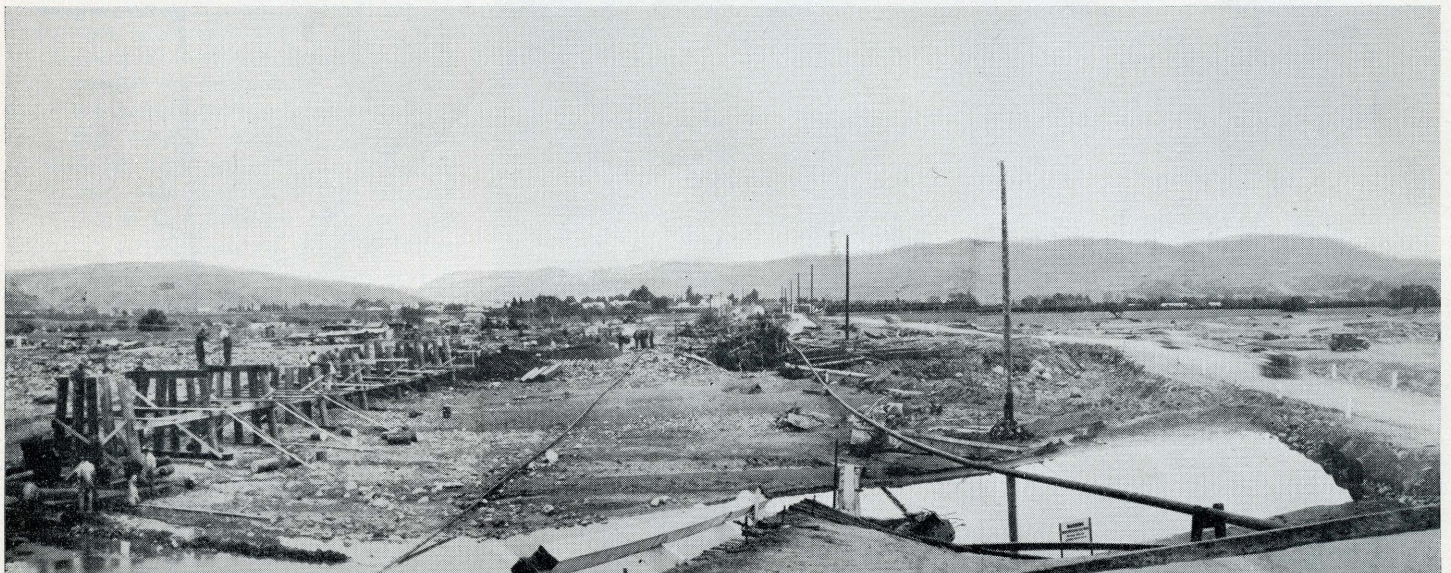
Sespe Creek swollen out of its banks by tributaries in a high mountain area of Ventura County cut a wide swath of damage as it swept across State Highway 79 near Fillmore. A county-built timber and concrete bridge and a paralleling railroad structure were washed away. A large section of highway was obliterated but a detour road shown at right was quickly built and opened.
