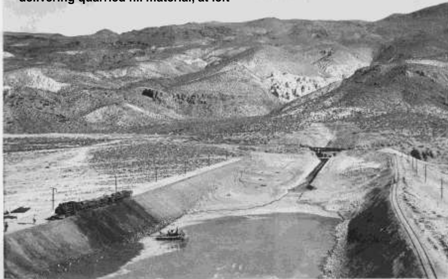
Haiwee Dam core pool, as viewed during construction in 1912. Note train delivering quarried fill material, at left
