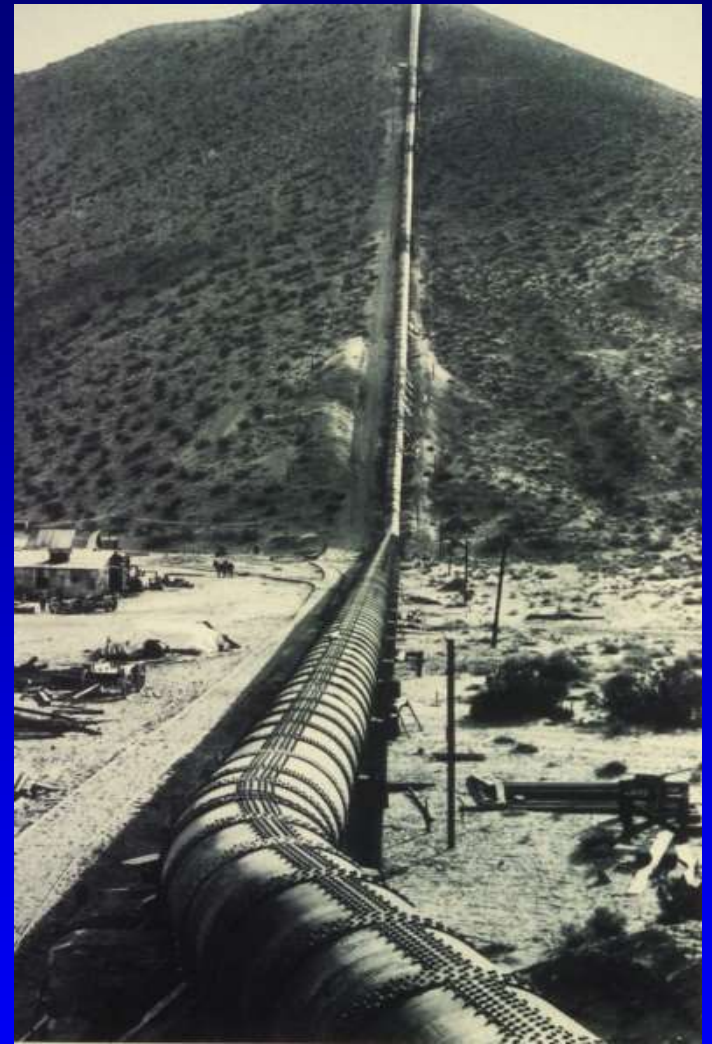
Right: Sag Pipe crossing Jawbone Canyon, dropping and rising 850 feet
