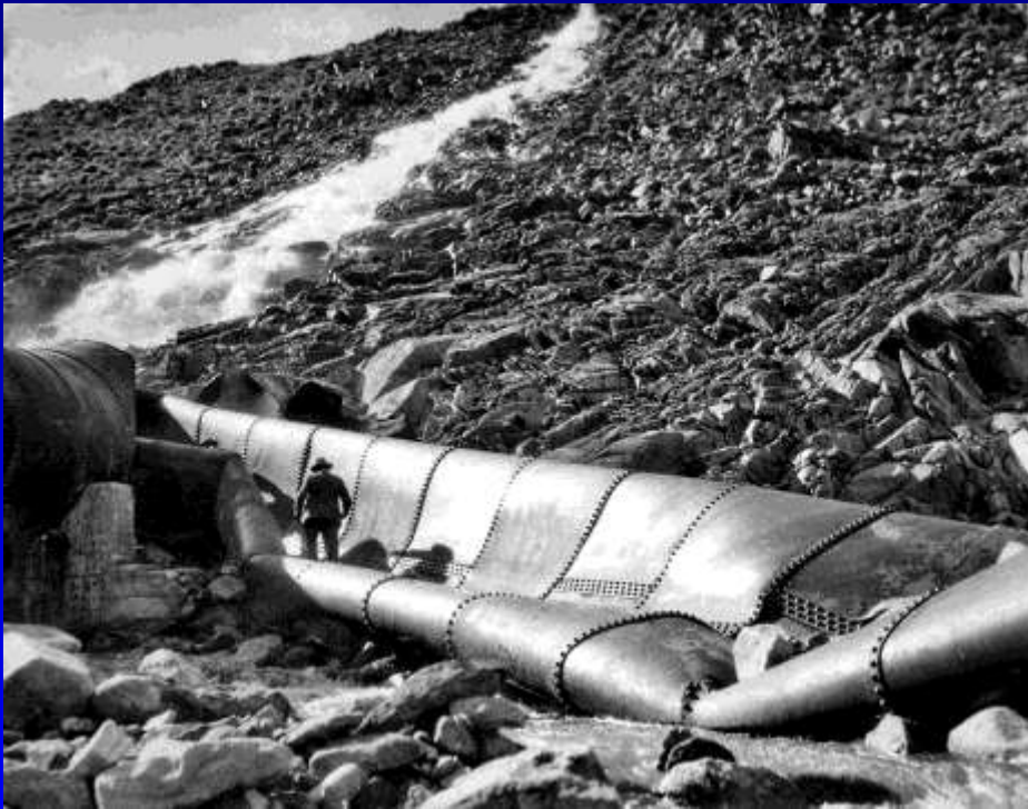
Above: Collapse of sag pipe in Sand Canyon in early 1913, after leaks undermined one of the footings, triggering implosion
