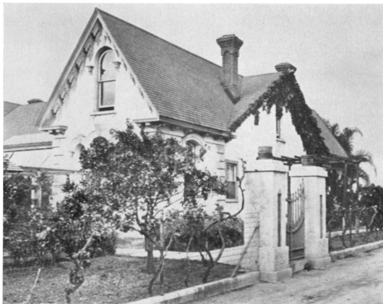
The old William Workman adobe at Puente. “. . . firm and sturdy to this day. . .”
