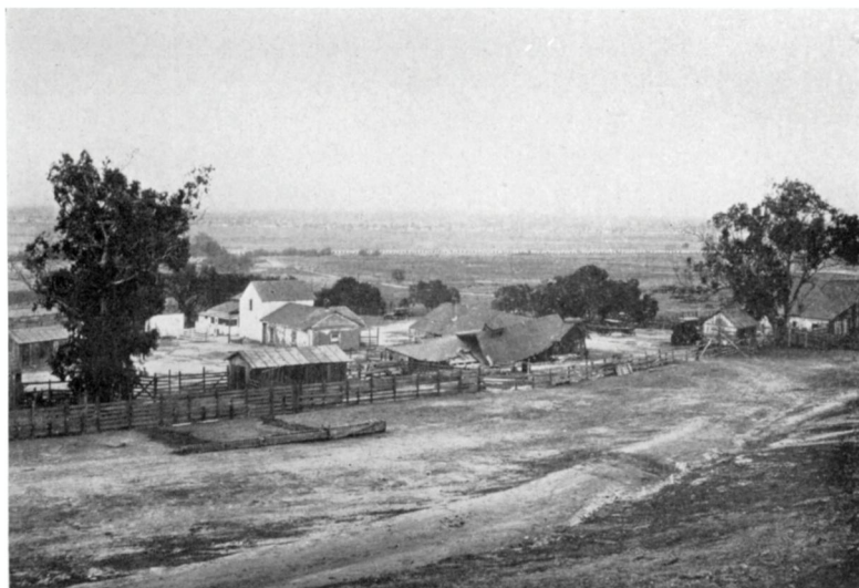
"Several adobe structures were reared during the long period that Rancho Ciénega was occupied as a rancho."
