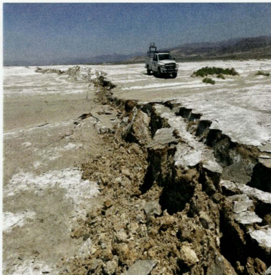
Zone of maximum surface displacement resulting from the 7.1 magnitude Searles Valley Earthquake. This was the largest earthquake to strike the Ridgecrest area during July 2019.
