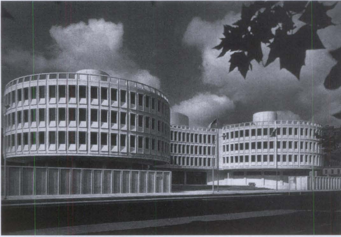
Figure 5. Following World War II, architects and engineers took advantage of improvements in concrete production, quality control, and advances in precast concrete to design structures such as the Police Headquarters building in Philadelphia, Pennsylvania, constructed in 1961. Photo: Courtesy of the Philadelphia Police Department.
