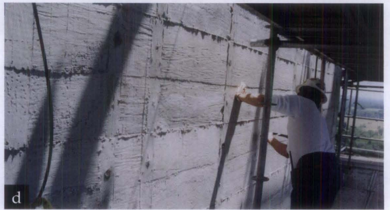
Figure 20. (a) The Jefferson Davis Memorial in Fairview, Kentucky, constructed from 1917–1924, is 351 feet tall and constructed of unreinforced concrete. The walls of the memorial are 8 feet thick at the base and 2 feet thick at the top of the wall. Access to the monument for investigation was provided by rappelling techniques, while ground supported and suspended scaffolding was used to access the exterior during repairs. (b) The concrete was severely deteriorated at isolated locations, with spalling and damage from cyclic freezing and thawing of entrapped water. In addition, previous repairs were at the end of their service life and removal of deteriorated concrete and failed previous repairs was required. Light duty chipping hammers were used to avoid damage to adjacent material when removing deteriorated concrete to the level of sound concrete. (c) Field samples were performed to match the color, finish, and texture of the original concrete. A challenge in matching of historic concrete is achieving variability of appearance. (d) The completed surface after repairs exhibits intentional variability of the concrete surface to match the appearance of the original concrete. Some formwork imperfections that would normally be removed by finishing were intentionally left in place, to replicate the highly variable finish of the original concrete. (e) The Jefferson Davis Memorial after completion of repairs in 2004. Photo e: Joseph Lenzi, Senler, Campbell & Associates, Inc.
