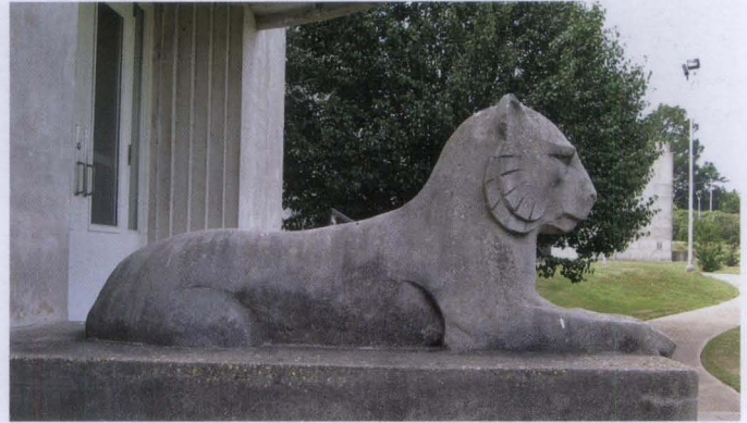
Figure 7. Detailed bas reliefs as well as sculptures, such as this lion at the Bailey Magnet School, could be used as ornamentation on concrete buildings. Sculptural concrete elements were typically cast in molds.
