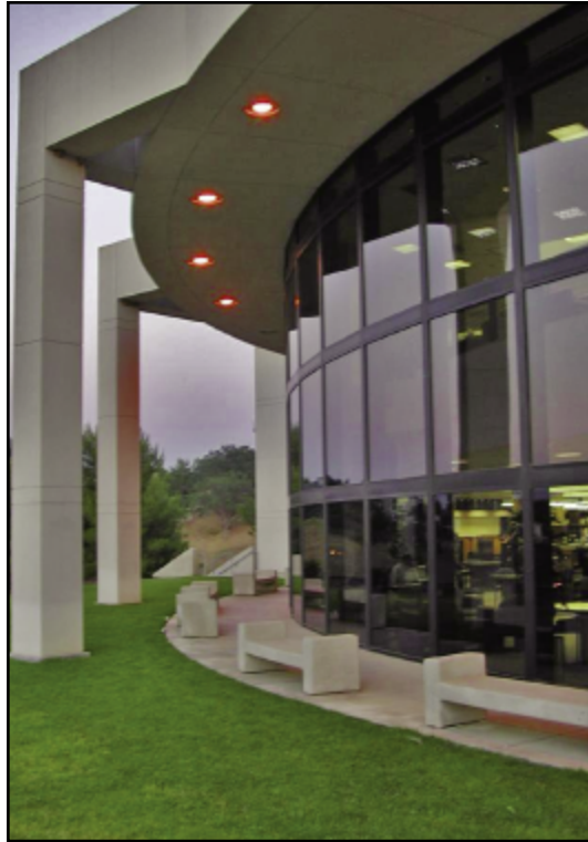
The hilltop Library’s two-story curved wall of glass provides visitors with a dramatic panoramic view of the Santa Clarita Valley.
