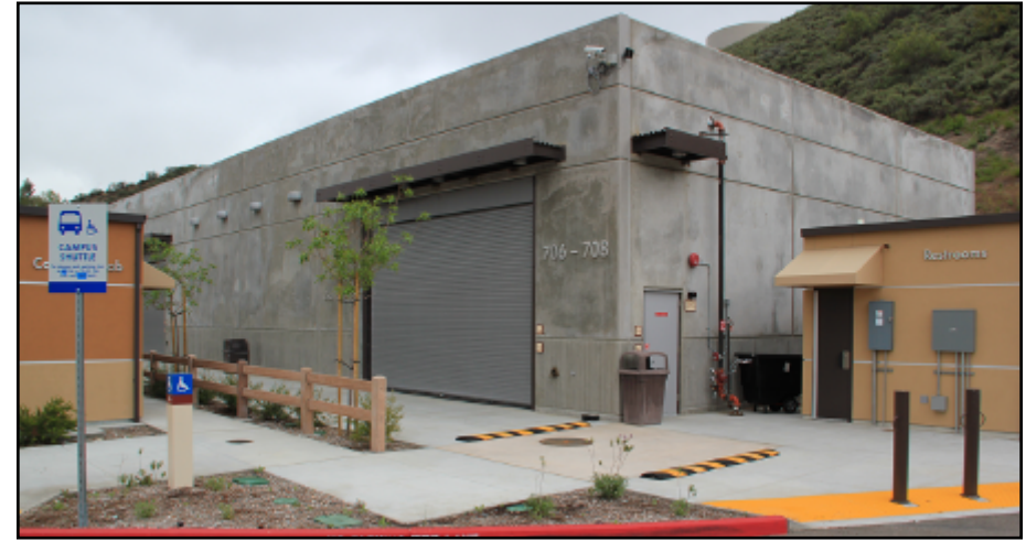
The Applied Technology Education Center, the first permanent building at the Canyon Country campus.
