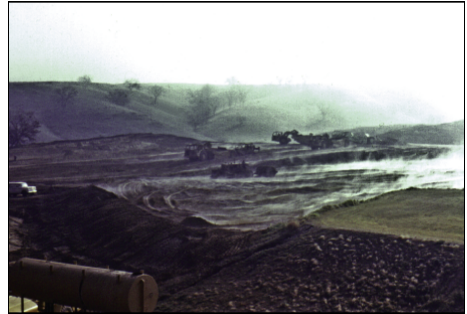
The hills south of Valencia Boulevard are graded to prepare for the construction of permanent campus buildings. The clattering steel behemoths kicked up an endless supply of dirt and dust at the nearby temporary campus.
