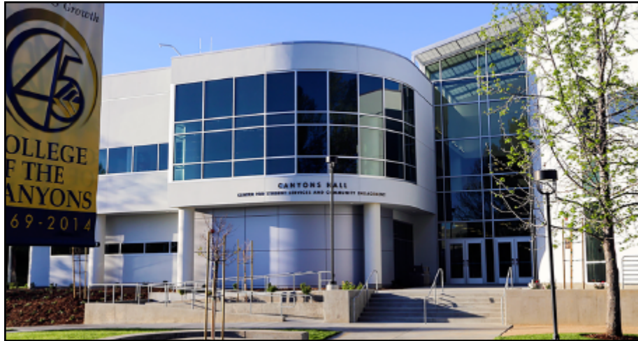
Canyons Hall, sitting at the main point of entry to the Valencia campus, is completed in early 2015.
