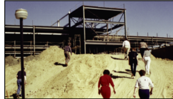
Employees check on the library's progress.
