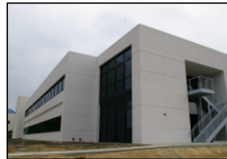
The Mentry Hall expansion project dramatically increased the building's teaching areas, and provided expansive common areas where students can study or relax (top).
