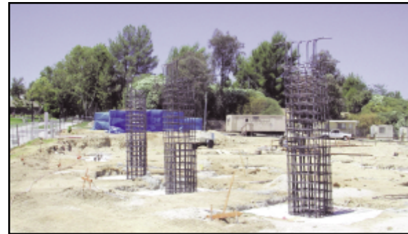
Construction of the Performing Arts Center begins.
