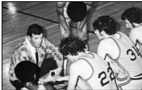
The Physical Education Center (top) is under construction in this view looking north. Already built and visible in the background is Cougar Stadium. Lee Smelser (above) was the college’s first men’s basketball coach.
