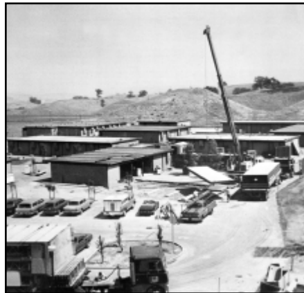
The athletic field, minus the stadium (top), and the modular buildings (above) being erected to create the temporary campus.
