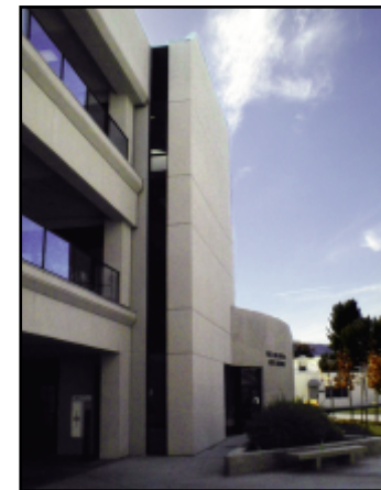
The steel framework (top) is pieced together to create the Media & Fine Arts Building (Mentry Hall, above).
