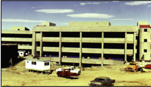
The Instructional Resources Center (IRC) under construction.
