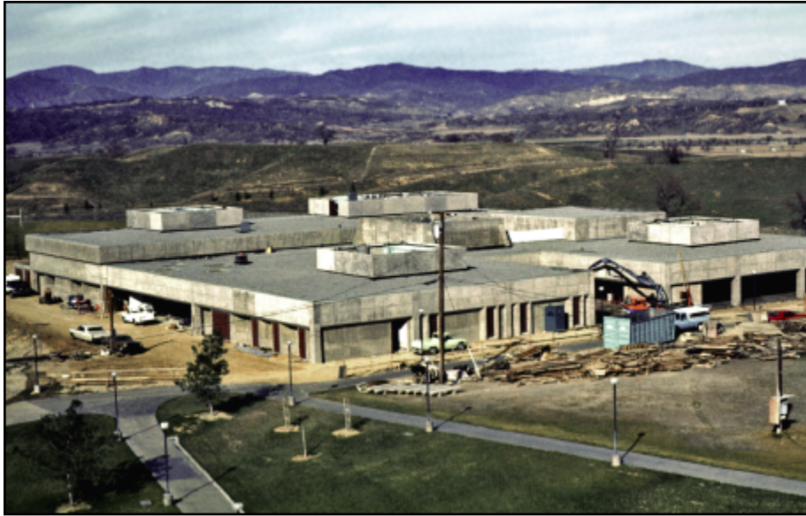
The Student Center is under construction in this view looking north.
