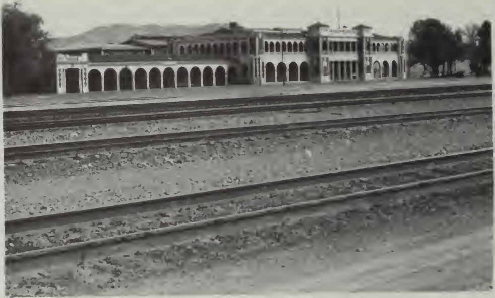
Figure 15. Casa del Desierto, the Santa Fe Harvey House at Barstow. W. E. Roberts
